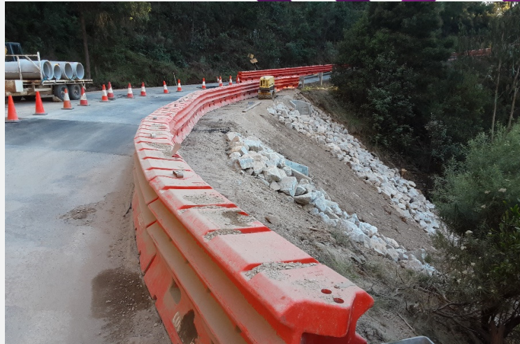
Landslip prevention works (now completed) on the Tawonga Gap Road
