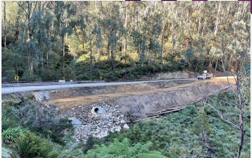
Works to extend existing culverts at Sassafras Gully
